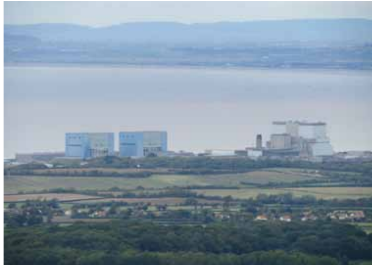
Hinkley Point nuclear power station from Higher Hare Knap Rory Walsh © RGS-IBG Discovering Britain
