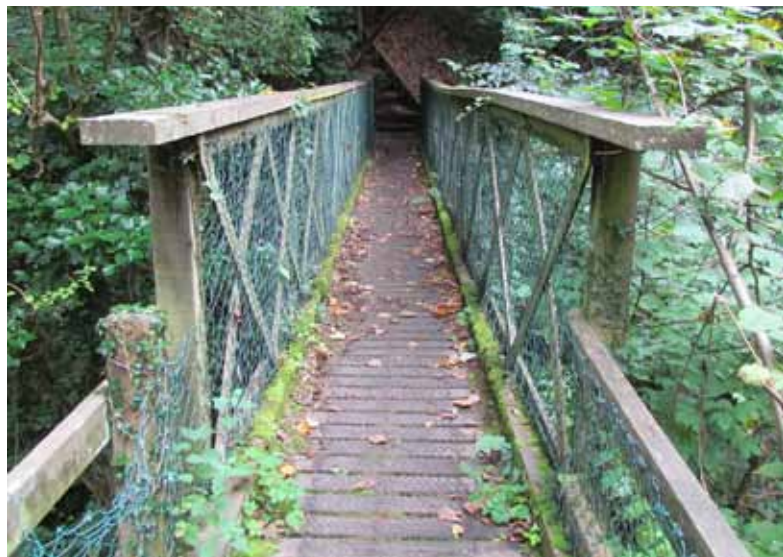
New bridge over Dorothy's waterfall, Holford Glen Rory Walsh © RGS-IBG Discovering Britain
